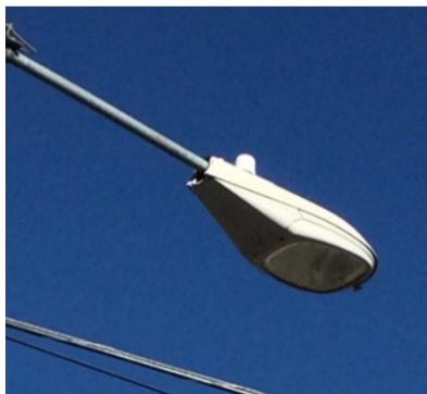
Figure 44: Non-LED Flat Fixture
