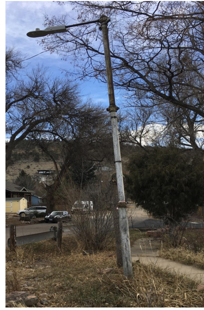
Figure 12: Steel Three-Tier Round Pole
