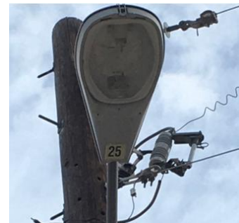
Figure 42: Non-LED #25 Fixture
