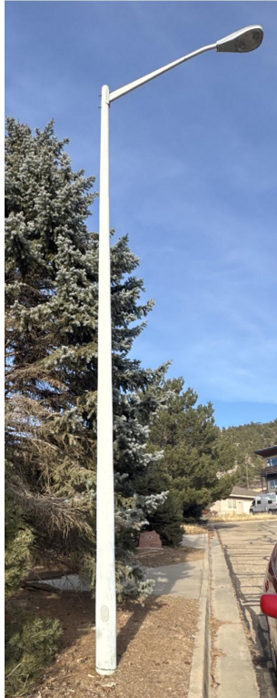
Figure 23: 20-Foot White Round Steel Tapered Pole
