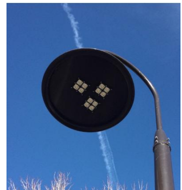
Figure 27: Main Street Alternative LED Fixture
