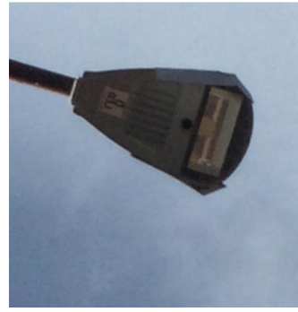
Figure 6: Fixture with Shield
