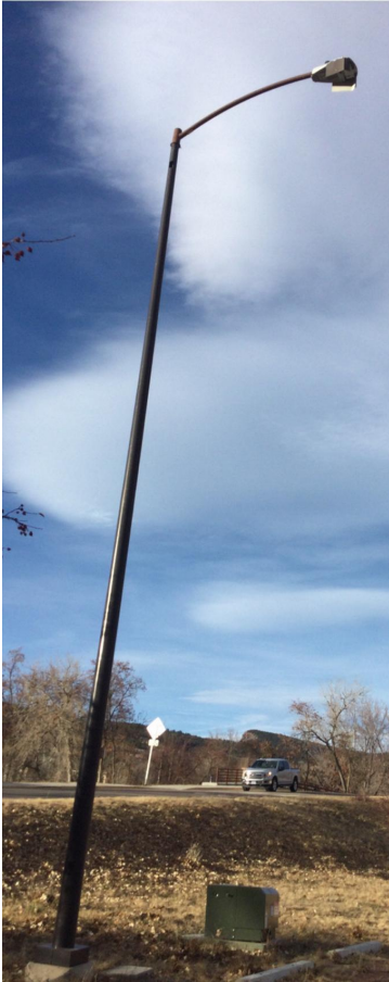
Figure 13: 32-Foot Round Steel Pole
