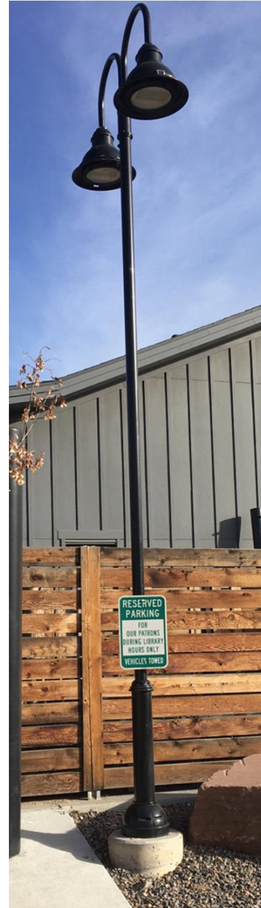
Figure 18: 15-Foot Tapered Round Steel Library Lot Pole Two Fixtures
