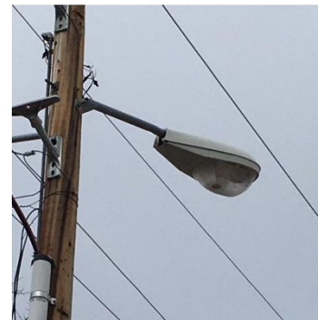
Figure 45: Non-LED Fixture
