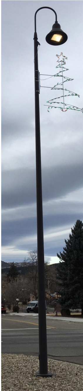
Figure 16: 24-Foot Tapered Round Steel Decorative Pole
