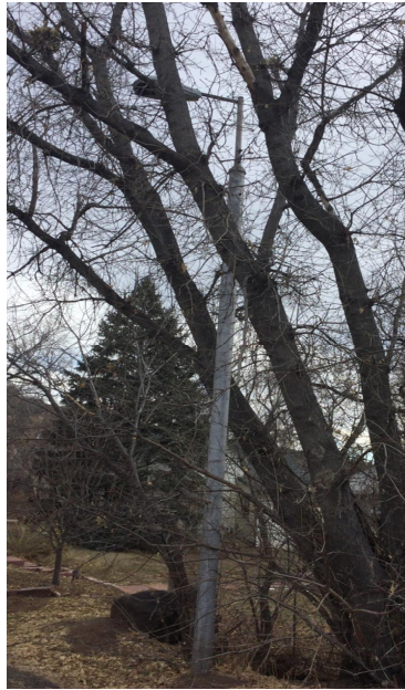
Figure 11: Steel Tiered Round Pole
