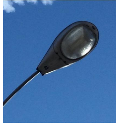
Figure 3: Non-LED Cobra Head
