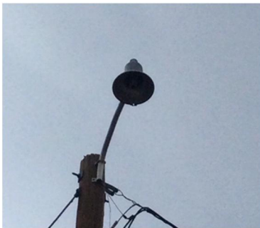
Figure 34: Traditional Non- LED Bell Fixture
