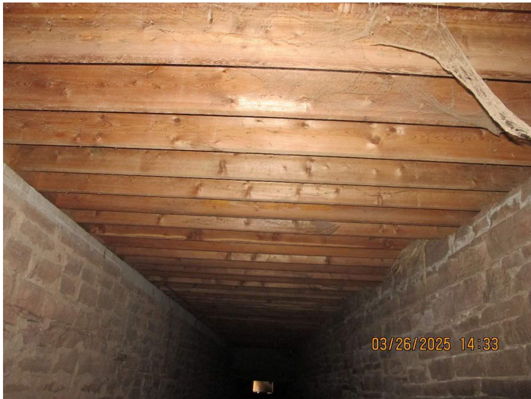
Photo E.6: Previous Repair Type PR6, South Culvert Station (S)9+71
