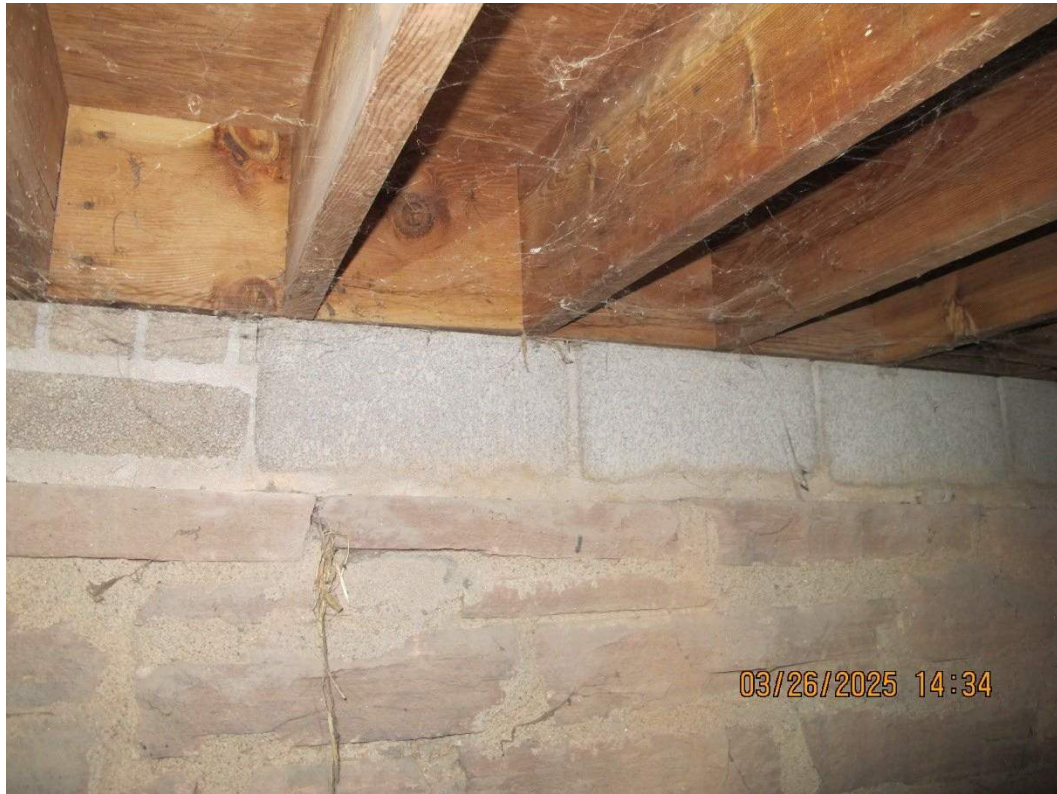
Photo B.13: Lid Construction Type L6 – Example 2
