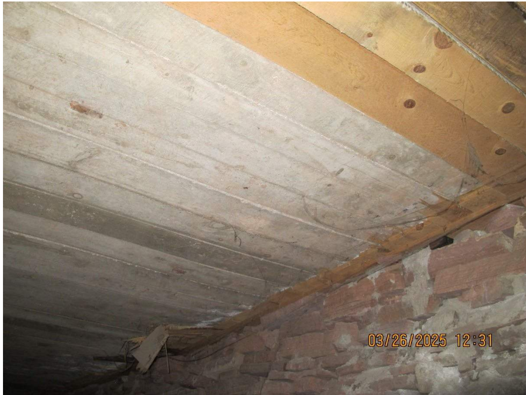
Photo B.7: Lid Construction Type L3 – Example 2
