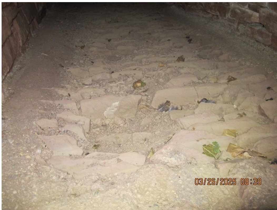
Photo B.30: Floor Construction Type F3 – Example 1
