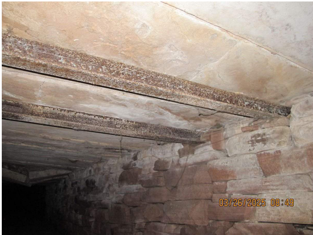
Photo E.2: Previous Repair Type PR2, South Culvert Station (S)1+35
