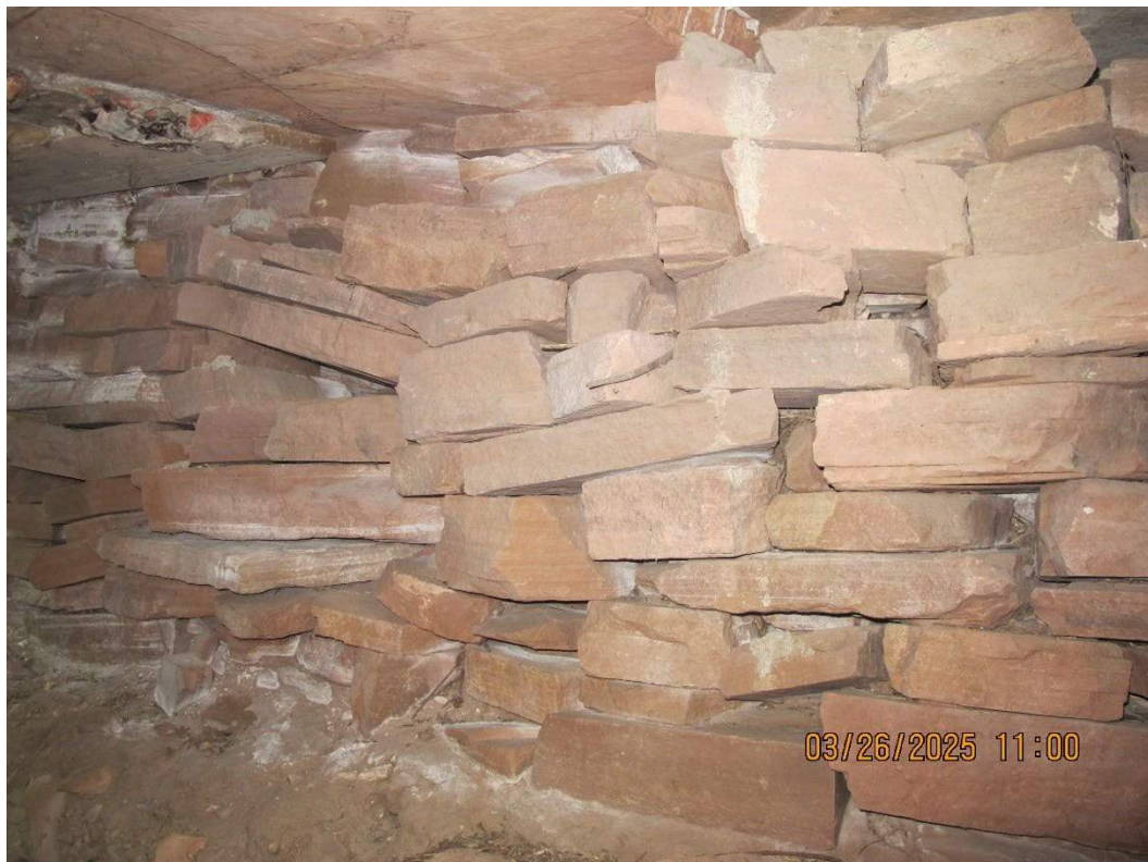
Photo B.18: Wall Construction Type W1 – Example 2
