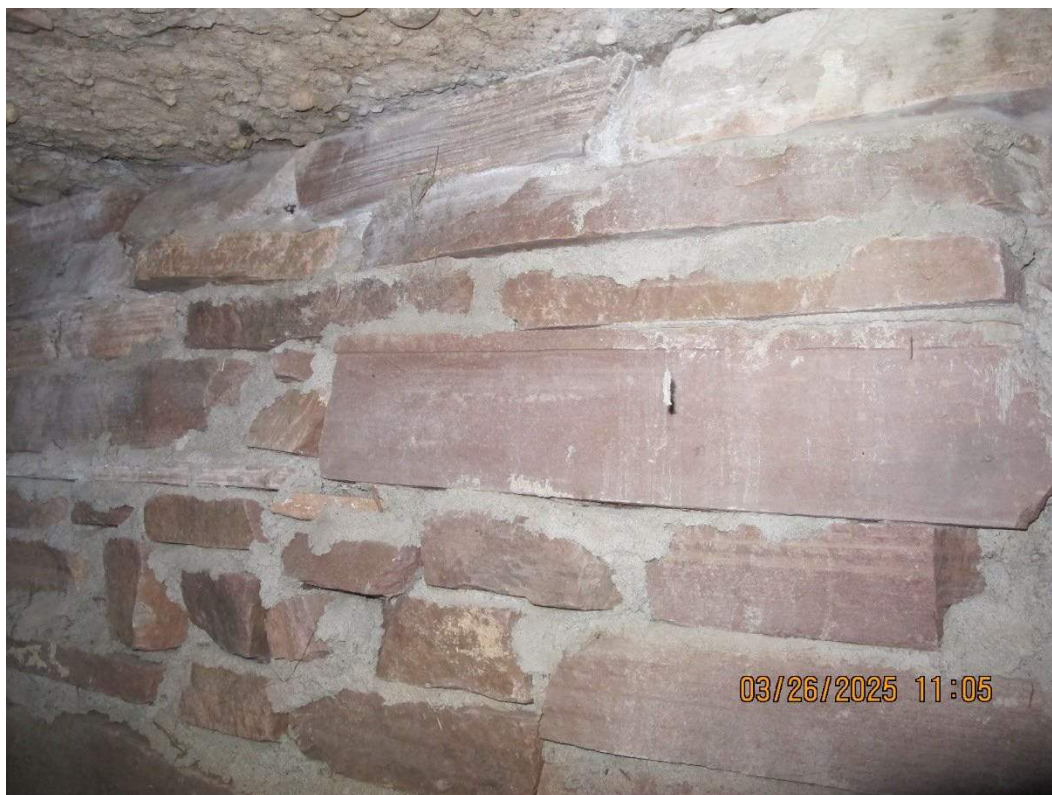
Photo B.19: Wall Construction Type W2 – Example 1
