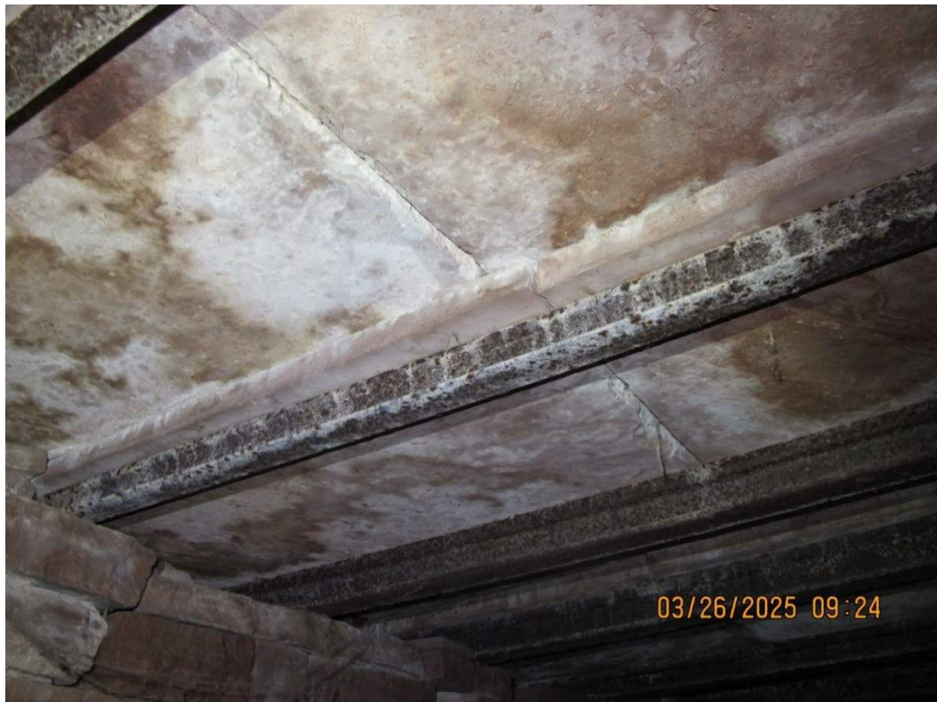
Photo B.2: Lid Construction Type L2 – Example 1
