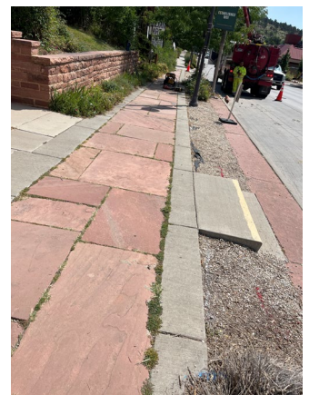
Sandstone sidewalk on Main Street.
