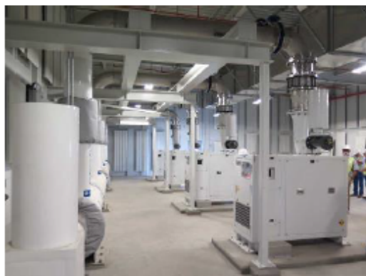
The MBR aeration blower building (ABB) includes acoustic panelling for blower noise abatement, making hearing protection unnecessary in the area.
