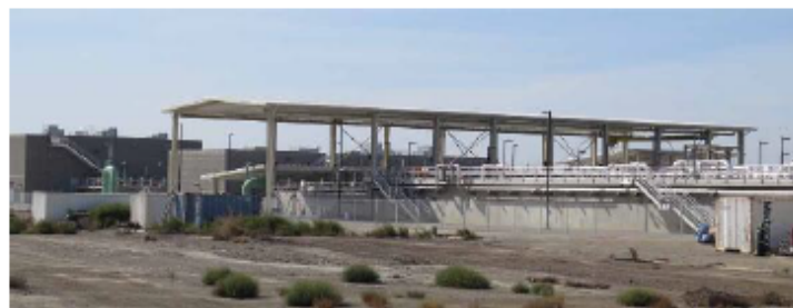
The Jennings STTF treats primary treated effluent for reuse using Biological Nutrient Removal (BNR) and MemPulse® Membrane Bioreactor (MBR) technology, followed by UV disinfection.
