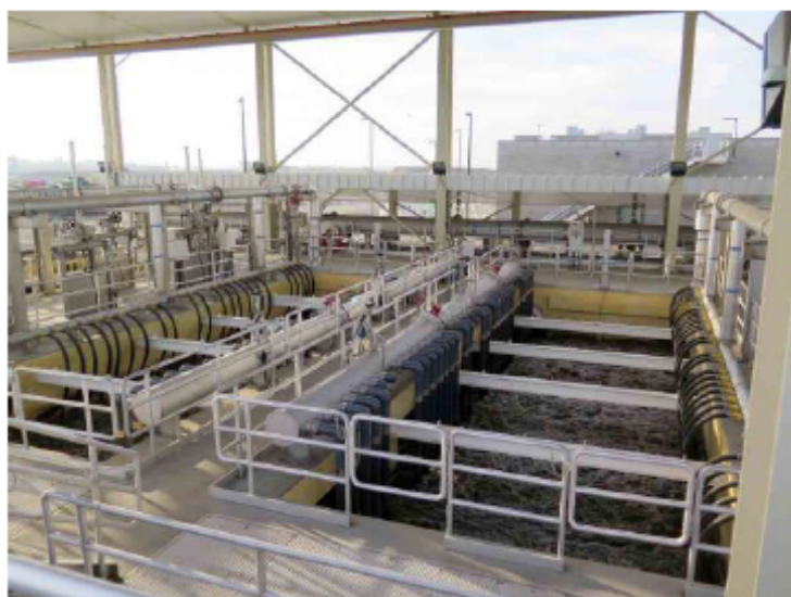
The six MOS cells at the Modesto plant each have provision for 34 x 16B40N MemRACK Assemblies with 28 racks fitted.
