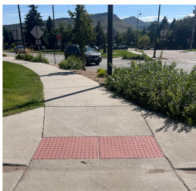
Curb ramp with detectable warnings and compliant landing on Old Main Street.
