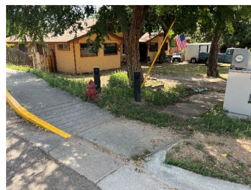
Curb ramp missing detectable warnings and compliant landing on Railroad Avenue.
