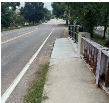
Missing sidewalk connection on 5 th Avenue bridge
