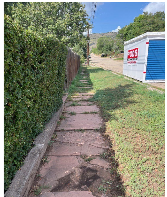
Existing sidewalk at 4 th and Stickney Avenue in need of major repairs, with obstructions if widening desired
