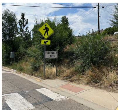
Curb ramp with detectable warnings on 5 th Avenue.
