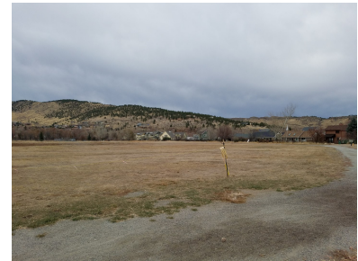
Red Hill Gulch Overflow Channel East would intercept flows before diverting runoff into Lyons Valley Park Subdivision
