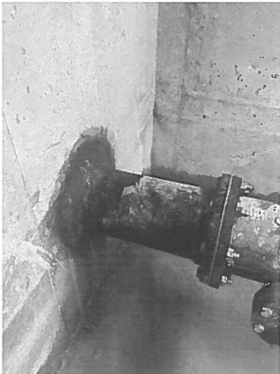
Image 5 – Seepage at east pipe penetration of PRV Vault 8
