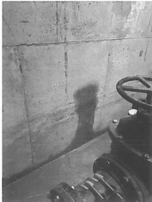
Image 6 – Seepage at south side of wall in PRV Vault 8
