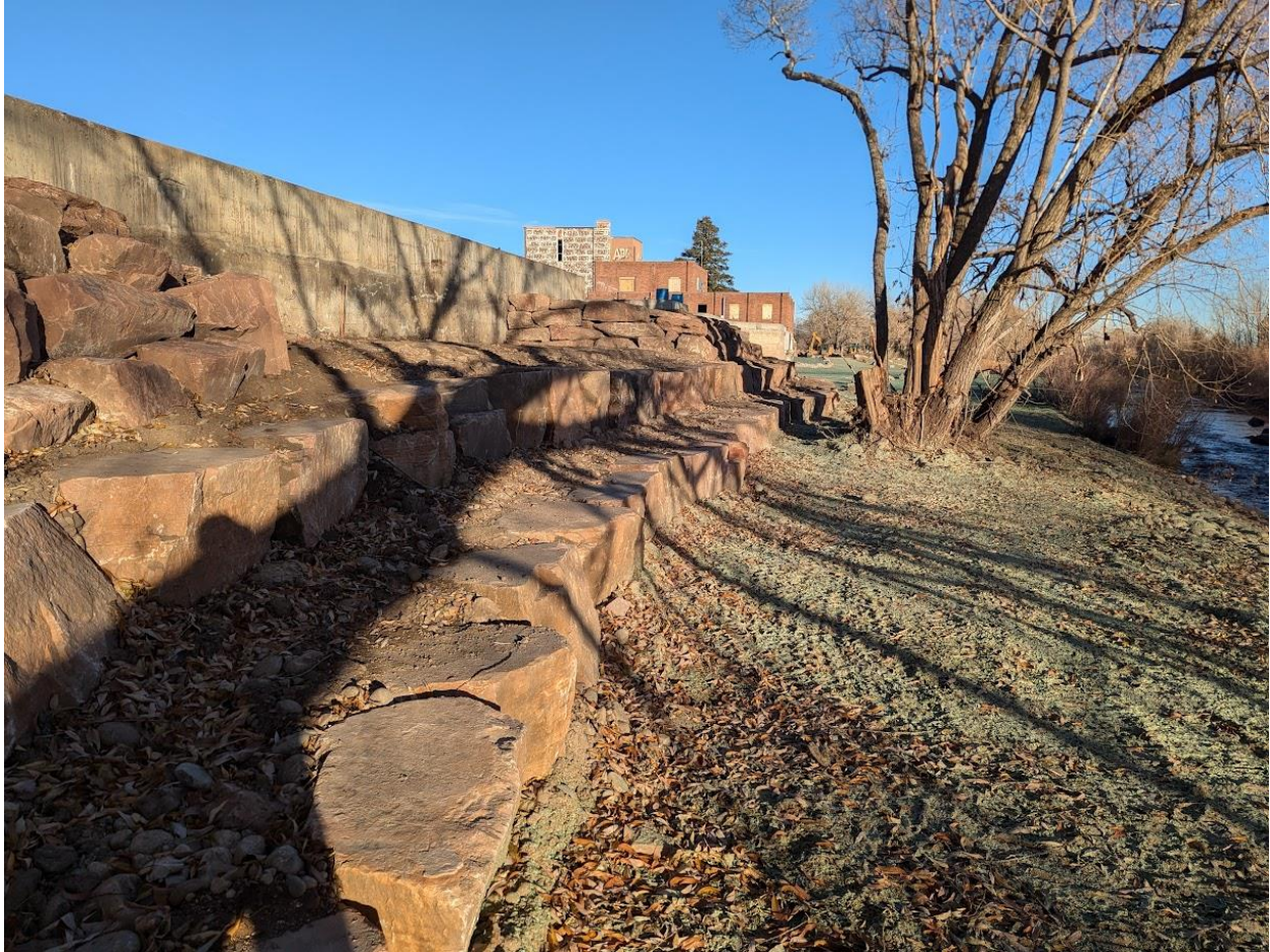
Figure 3 Final terraced boulder revetment with recessed upper row.
